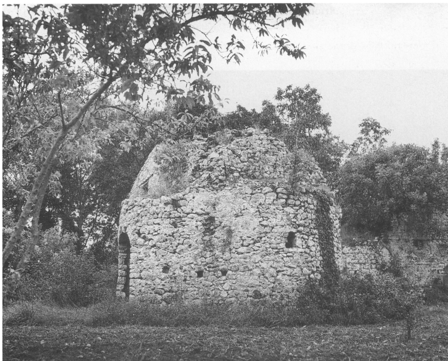
a General view of the triconch chapel showing the east lobe with the central window and the south lobe with the phase 3 door, note the putlog holes (Photo Ray Manley)
