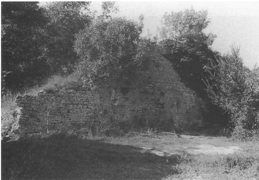
a Photograph of the east side of the south pier showing the incline of the early medieval bridge. (Photo: Richard Hodges)
